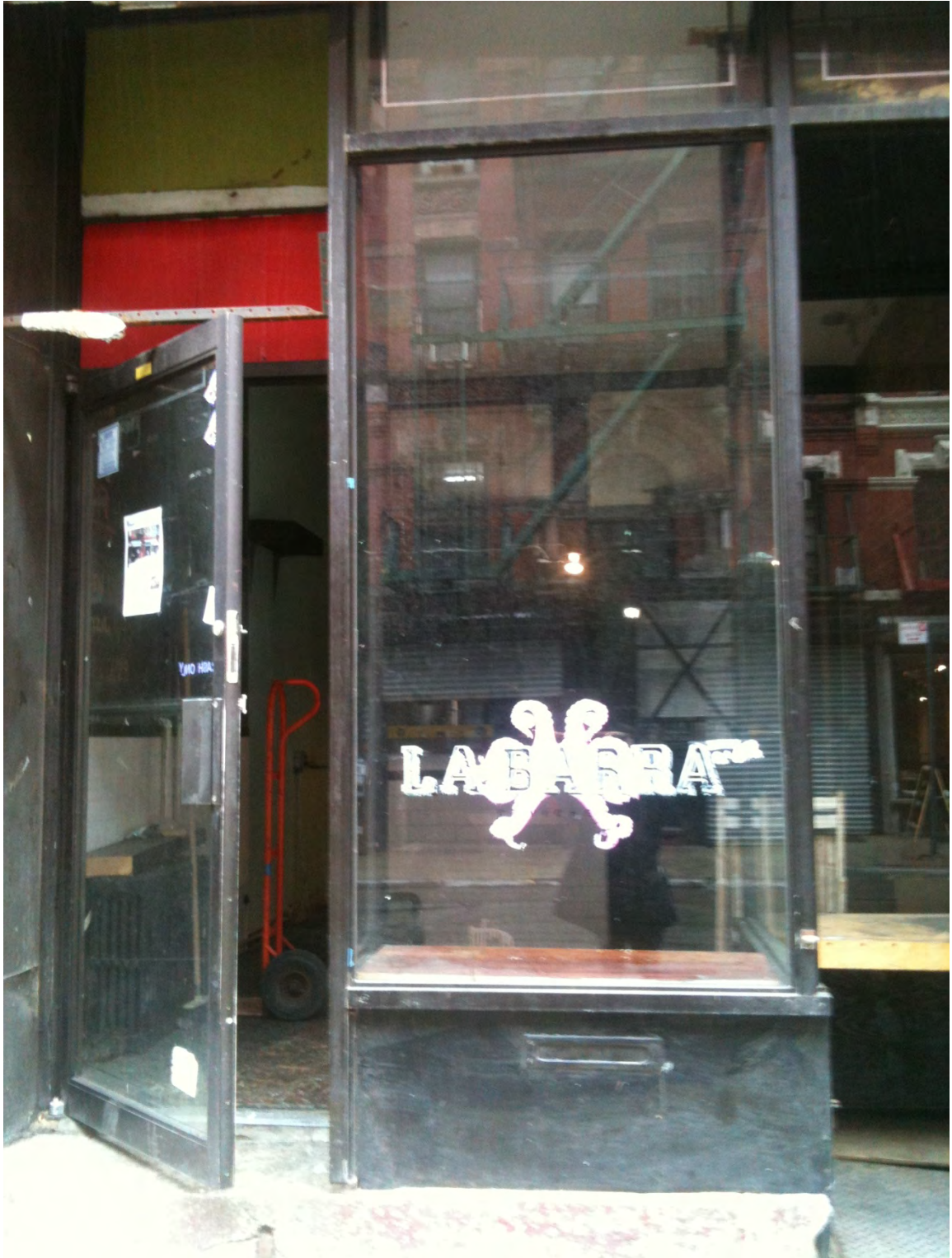
View of the outside storefront at 250 Broome Street ( in progress )
